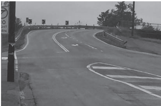
The Weston Bridge, NSW.
