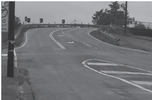
The Weston Bridge, NSW.
